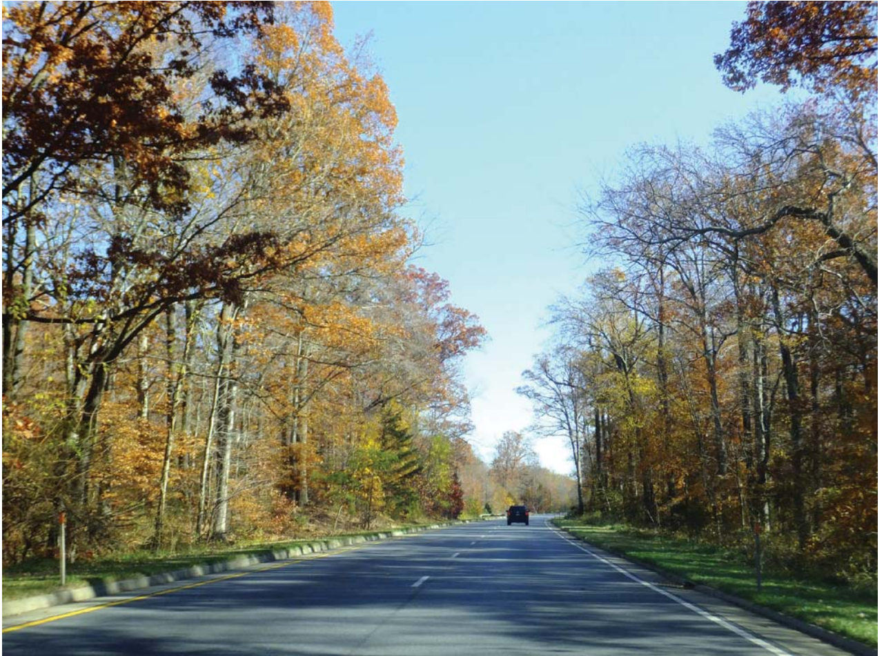
Suitland Parkway National Capital Parks - East
