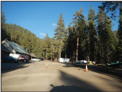
Parking area was not rated because it was under construction.
